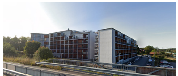
Recent bloc development, Trunstavägen
